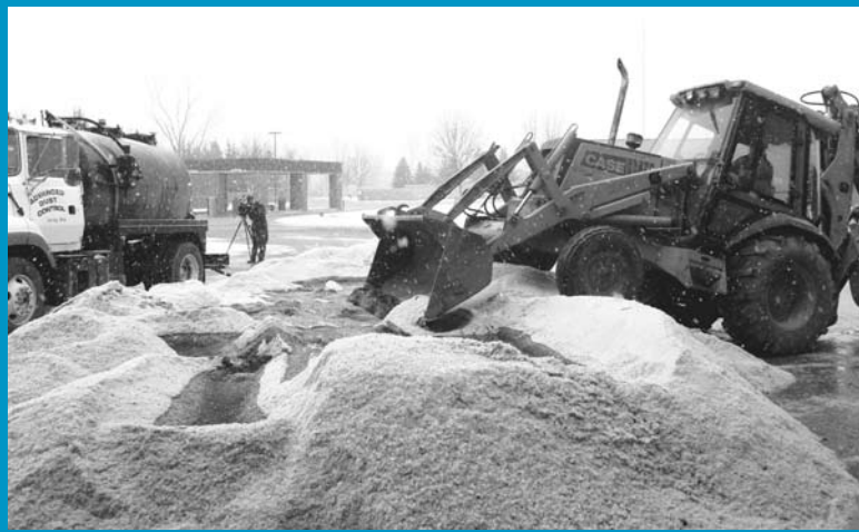
The de-icing liquid is shown being mixed in with the road salt.
